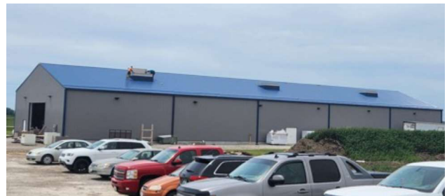
Figure 6: Warehouses for materials storage built at the Homes for Iowa building site
