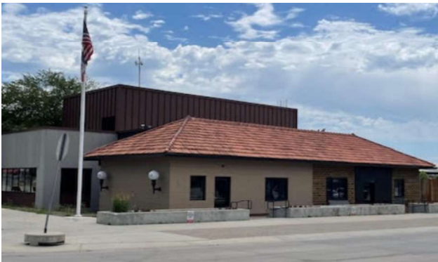
Figure 32: Exterior and interior work completed on the Iowa State Fair Police Headquarters building
