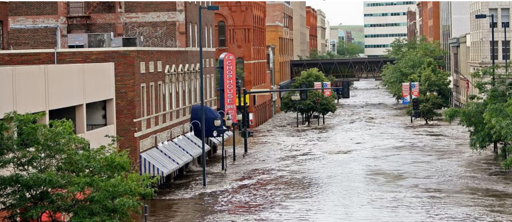
Flooding in downtown Cedar Rapids in June 2008.
