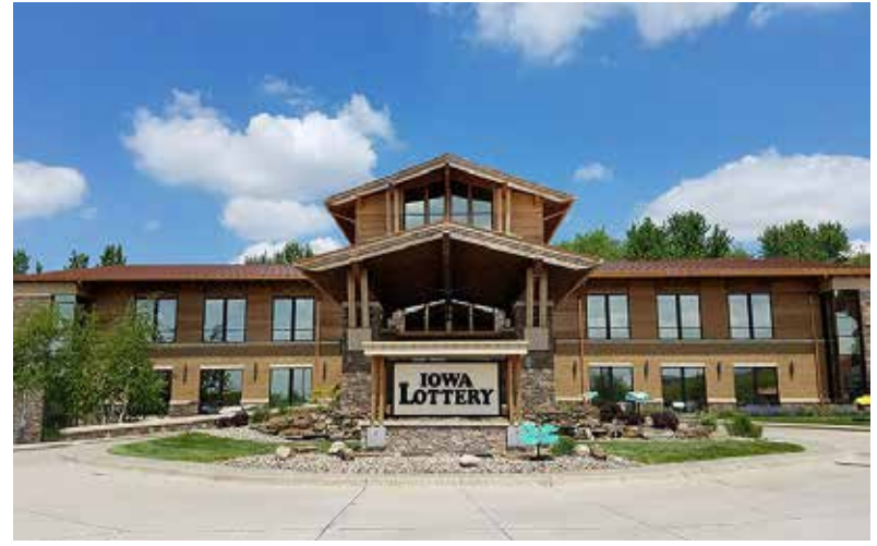
Iowa Lottery headquarters is located at 13001 University Avenue in Clive.
