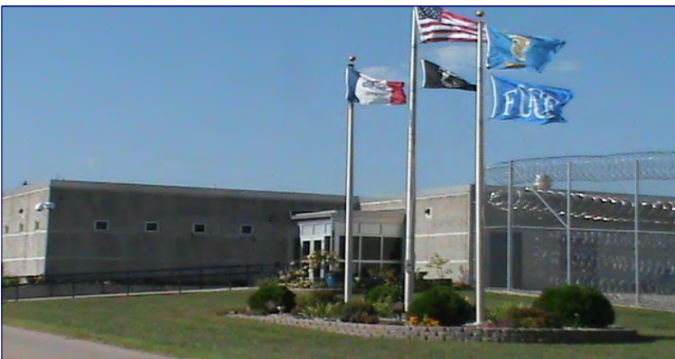
Fort Dodge Correctional Facility, Fort Dodge
