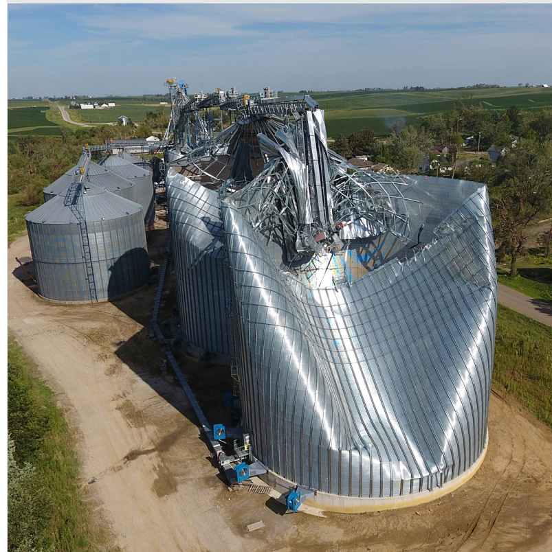
Tama County grain bins collapsed in the derecho storm. Photo: Kip Ladage, Bremer County Emergency Management
