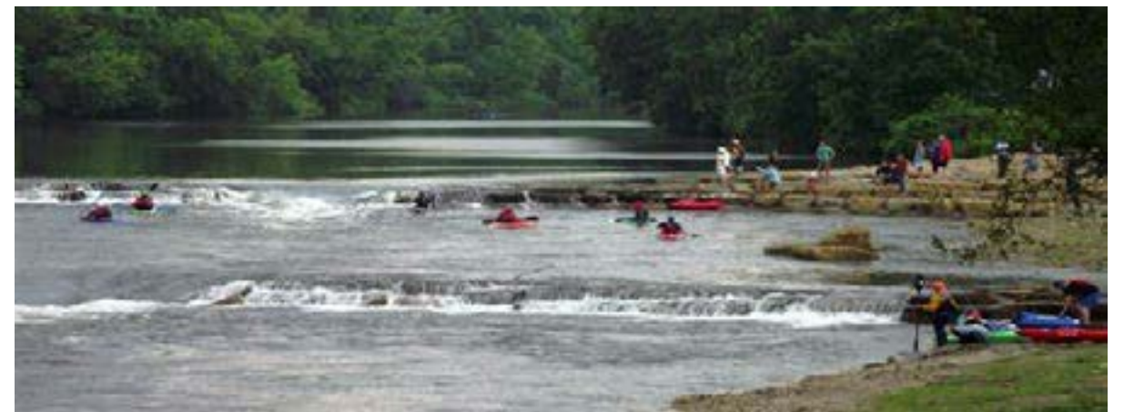
Dam converted into a whitewater opportunity with improved fish passage.
