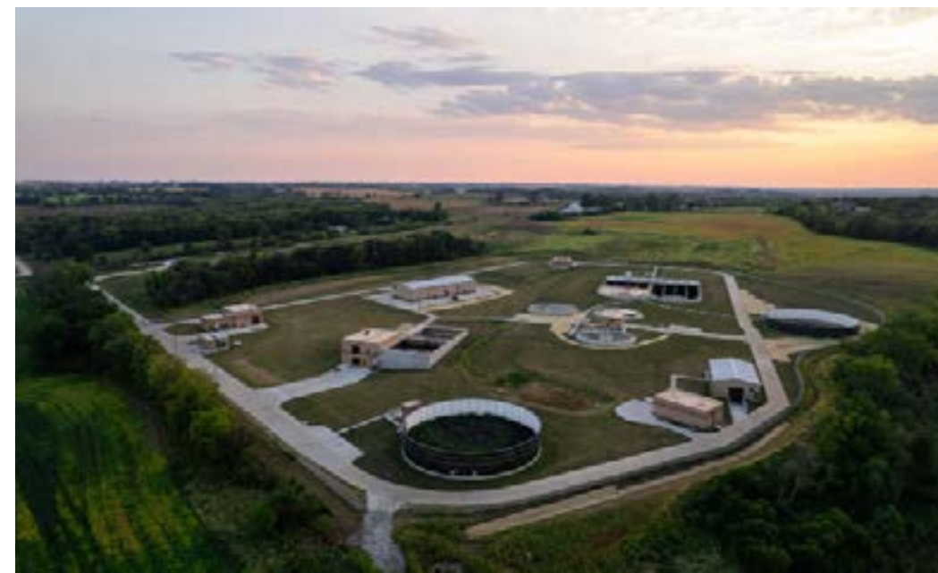
The new Indianola Water Resource Recovery Facility, commissioned in 2022, will replace the aging wastewater treatment plant, reduce the nutrient (nitrogen and phosphorus) loads in to the Middle River to meet the goals of the Iowa Nutrient Reduction Strategy. This new facility has the capability to manage peak wet weather flows utilizing the treated wastewater to irrigate the nearby Indianola Country Club golf course.
